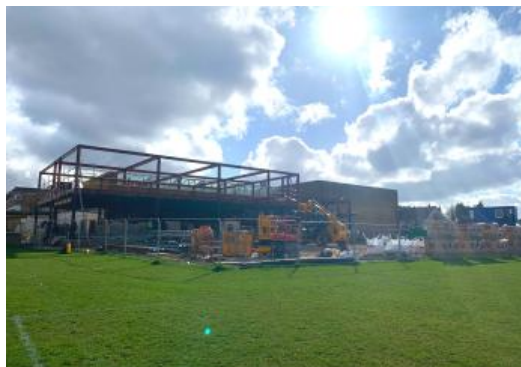
Building work continues at a pace!
